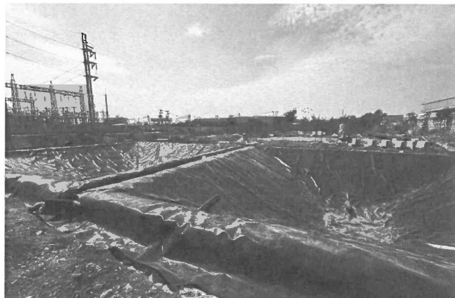
Install HDPE Sheet
