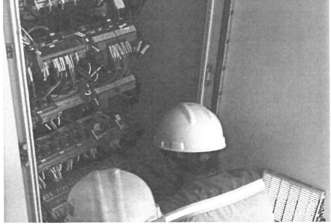
Cable Terminate for Engine Control Panel
